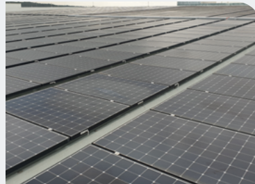
Installation of Canteen Solar Roofing
