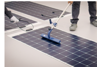
Installation of Maxeon Air solar panels
